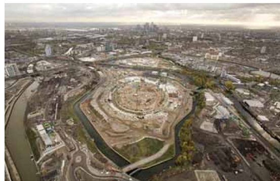
Progress at Olympic Park (Photo courtesy ODA)
