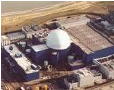
Sizewell B Nuclear Power Station
