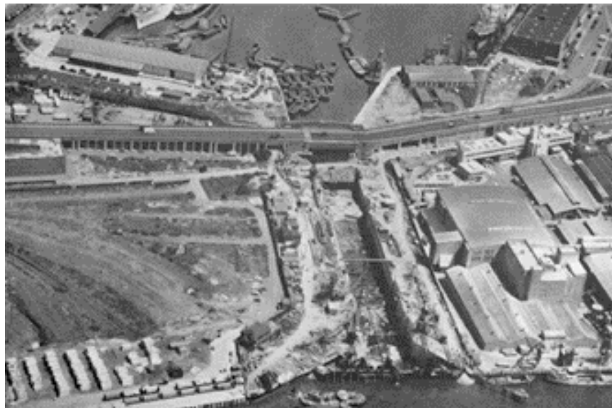
Aerial view of site at high tide in the river Thames during the period of peak construction.
