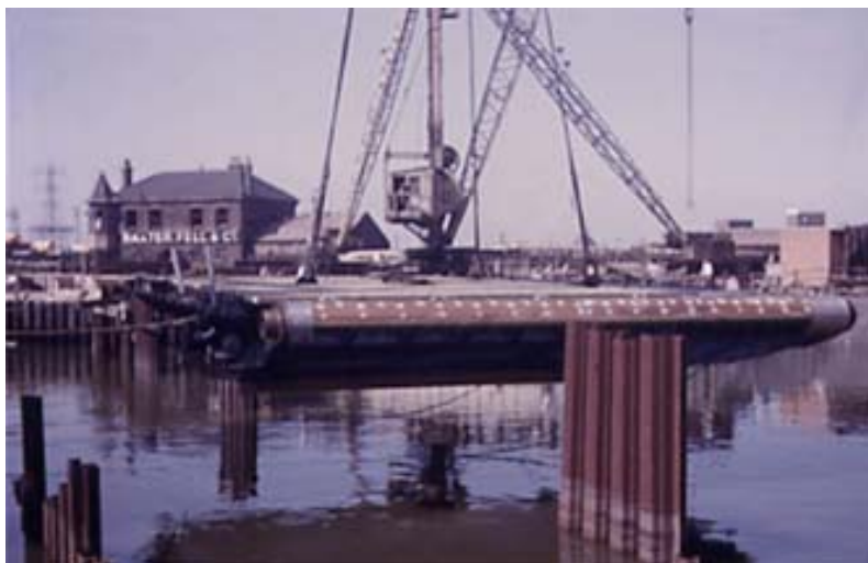
Lifting the 120-ton lock gate leaf into position.
