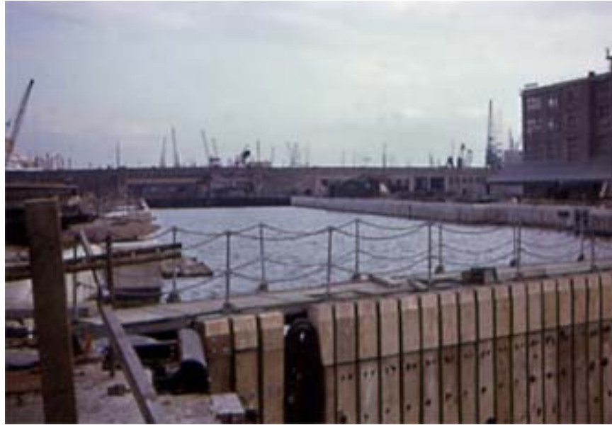
Finished lock filled to brim and under test.
