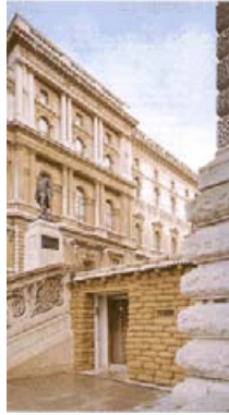
Figure 20.1: Storey's Gate Entrance to Churchill's Bunker
